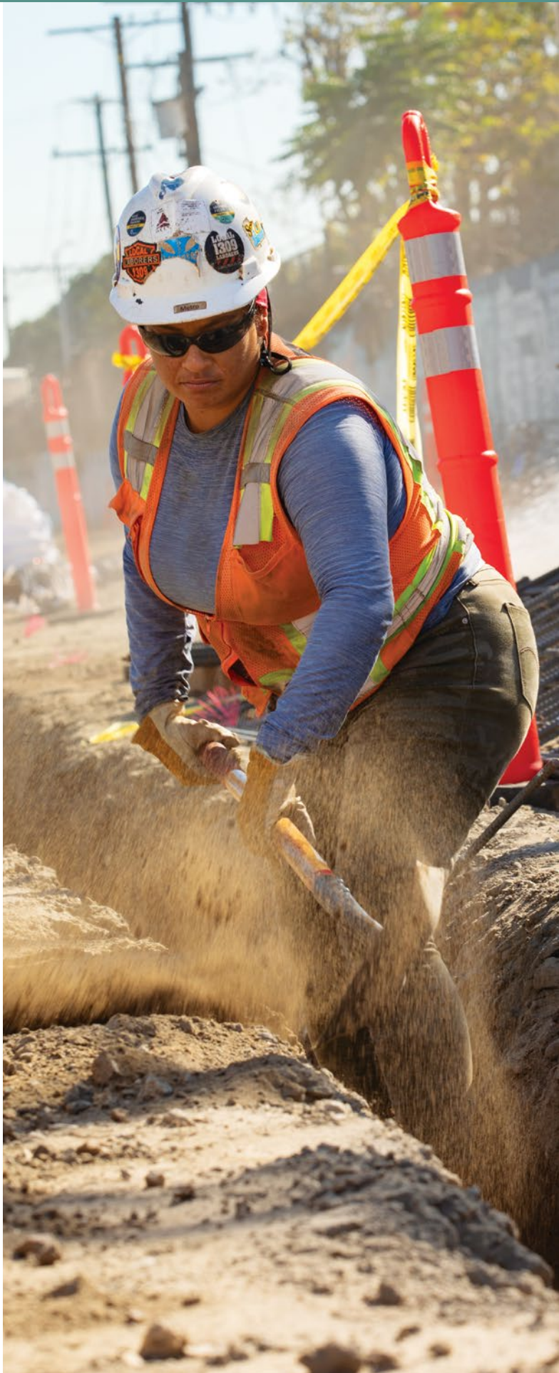
Cover: Red Line Construction (1993). Image from the Metro Art exhibition Ken Karagozian, Deep Connections , previously on view at the Union Station Passageway Art Gallery.
