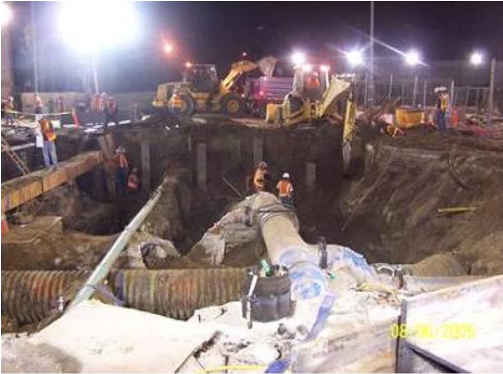
Gold Line Eastside Extension – excavation for south row of piles at Soto Station
