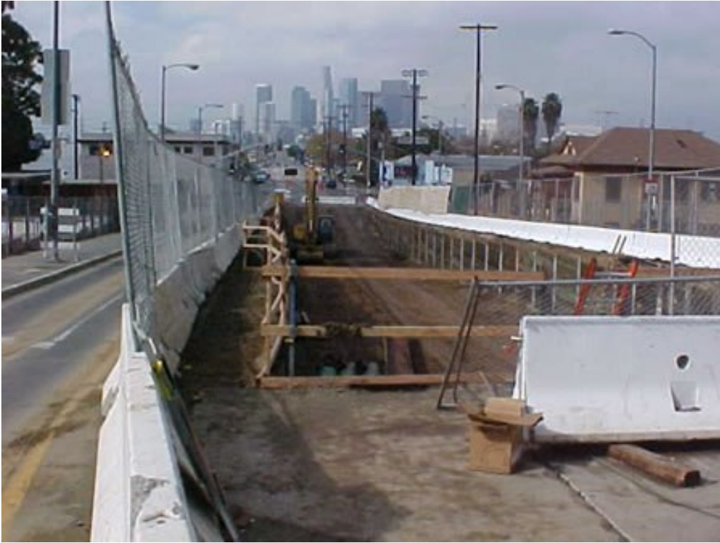
Gold Line Eastside Extension – West Portal excavation
